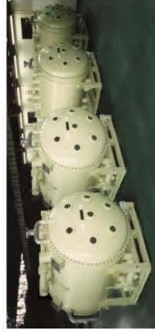
Drinking Water Treatment (31.0 kg-O 3 /h x 4 sets)
