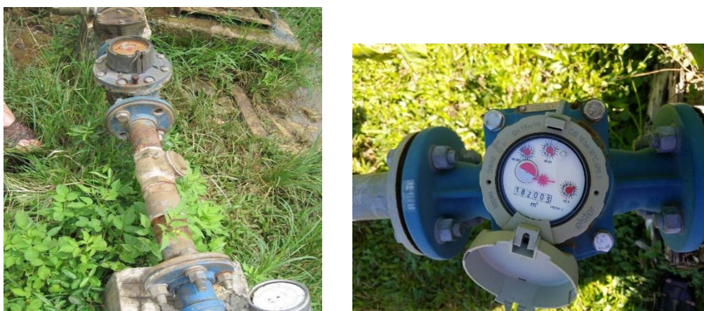
Photo 2.1 Malfunctional Flow Meter
