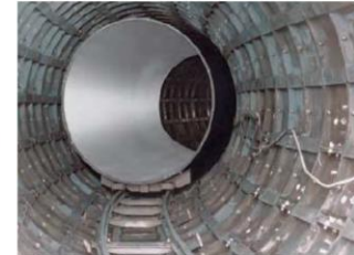
[Sheath pipe for water supply] Small Section Shield + Ductile iron pipe (earthquake-resistant pipe)
