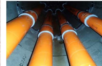
[Sheath tube of electrical cables] Small Section Shield + power cable tube
