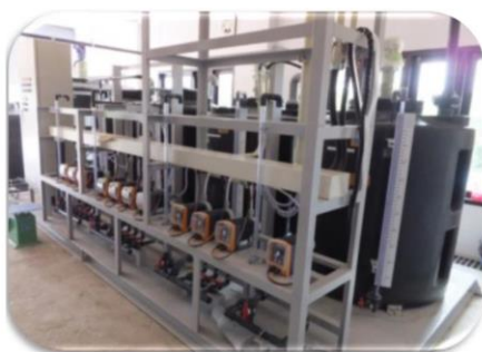
Chemical dosing pump (Aluminium, Chlorine, polymer)
