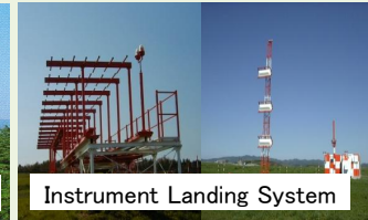
Instrument Landing System Transmits landing course to aircraft by radio wave
