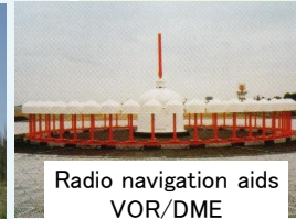
Radio navigation aids VOR/DME Provides information of direction and distance to aircraft
