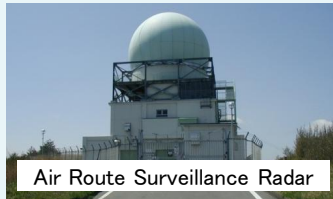
Air Route Surveillance Radar Detects positions of flying aircraft
