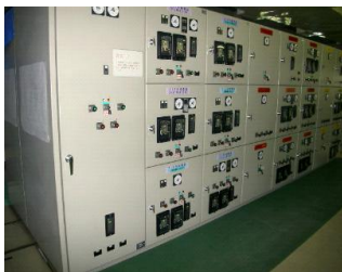
Unit Substation
