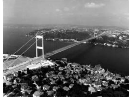
144. (2 nd Bosphorus Bridge, where work has begun on earthquake strengthening (Turkey))
