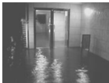
Scene of flooding brought on by torrential rains (Suginami Ward, Tokyo)
