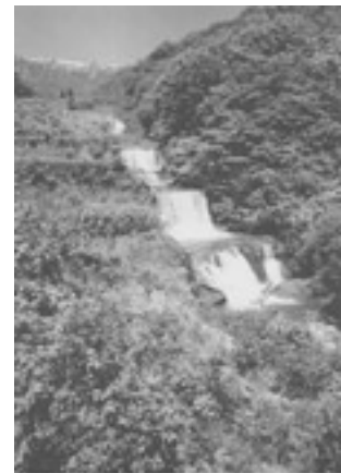
Bannai River Sabo Dam, registered as a designated tangible cultural property (Niigata Prefecture)
