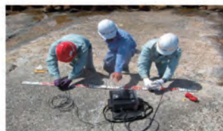
護岸の点検・補修
