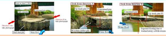
Probable causes : It is highly probable that the accident occurred as the 2nd axle in the rear bogie of the 3rd vehicle had derailed to right because the train was running on the track on the bridge significantly deformed by the subsided and tilted pier, after that, the derailed axle restored in the level crossing while passed as being derailed.
