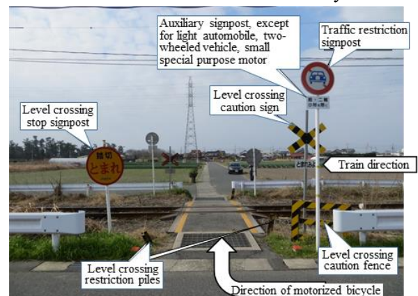
<Status of Niiya No.3 level crossing viewed from the entered side of the motorized bicycle>
