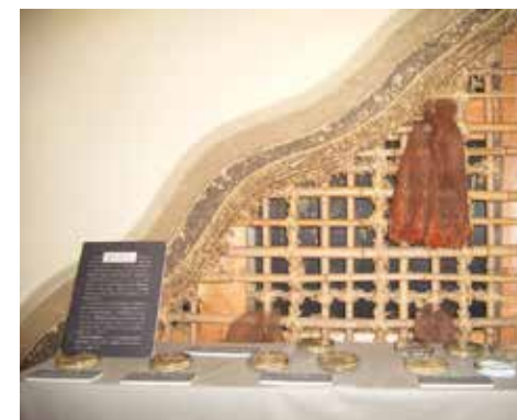
To build mud walls, assemble the komai first and then plaster mud in several layers.
