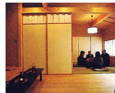
Interior doors which incorporate muso (window made of narrow boards connected on two rails each of which slides for opening and closing) on the top for interior ventilation
