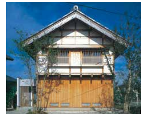
External wall finished with plaster coat at the top and boards on the bottom where the wall is exposed to rain.
