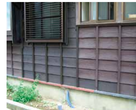
Partially replaced boarding and repainted so the repaired part is not conspicuous. (Washima, Niigata Prefecture)
