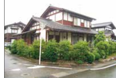
Sloped roof with tiles (Toyama Prefecture)
