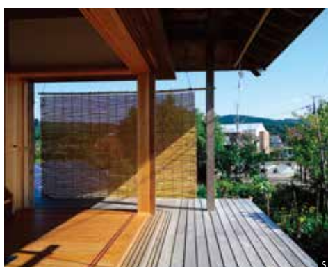
Sunscreen hung under an eave; would be more durable if hung a little more inward.
