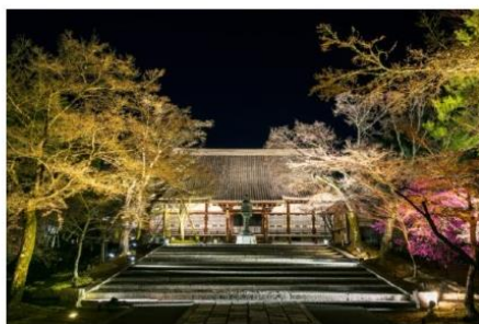
The kondo (main hall), illuminated at night
