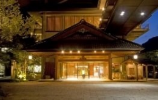
Large-scale renovation of accommodation facilities
