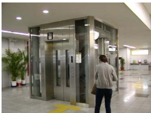
Installation of elevators
