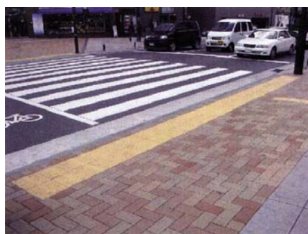
Improvement of level differences and slopes on sidewalks and the installation of guide blocks for visually handicapped people
