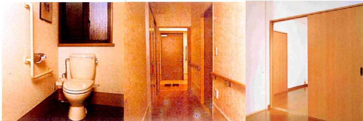
Installation of handrails
