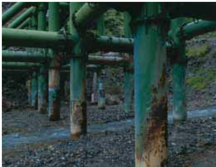
鋼鉄製の砂防おん堤
