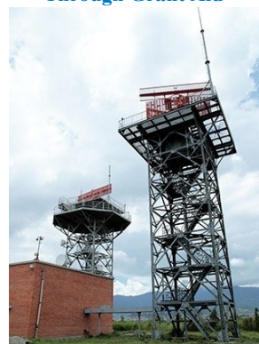
Figure 4-18 Construction of Radio Facilities Through Grant Aid
