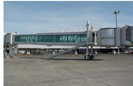
Full Flat Floor Type PBB Exterior View
