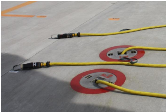
Pits for electric power
