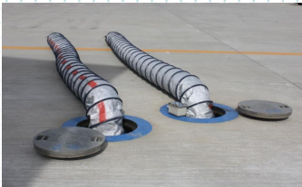
Pits for air-conditioning air
