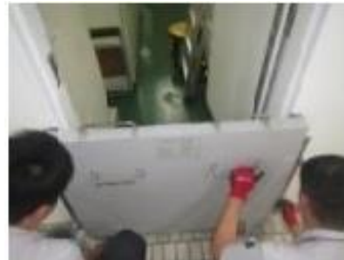
On-site response training (installation of waterstops) (Nagasaki Airport, May 2019)
