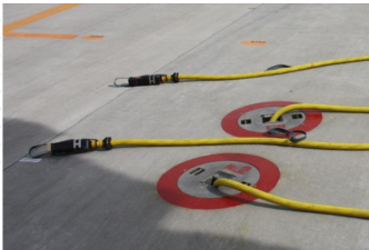
Pits for electric power
