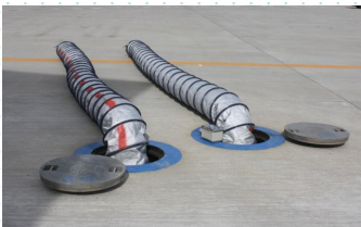
Pits for air-conditioning air
