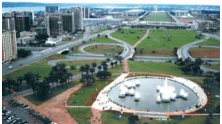
The public office area and the area where the wings meet the body, seen from the TV tower
