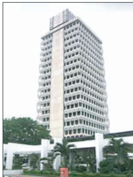
The office building adjacent to the Parliament House (Kuala Lumpur)
