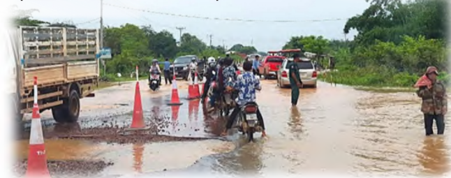
Road condition after squall, October 14, 2020
