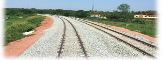
Circular railway track
