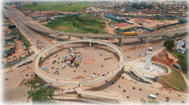
Three steel pedestrian bridges (circular pedestrian bridges)
