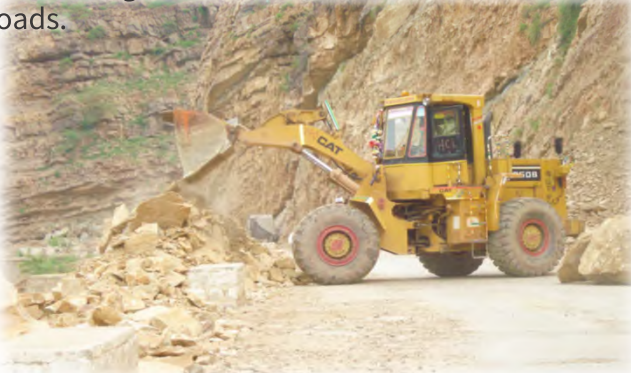
Road restoration work using wheel loader
