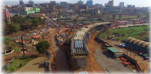
Construction scene of a viaduct
