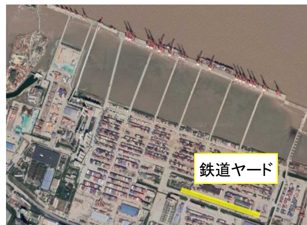
寧波港 (Beilun International Container Terminal)
