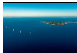
Block Island Wind Farm
