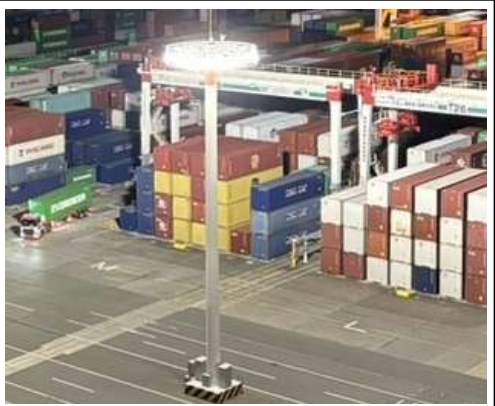
Conversion of 10 Yard Lighting Units to LED
