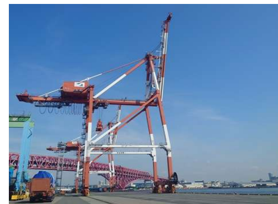
STS with inverter system
