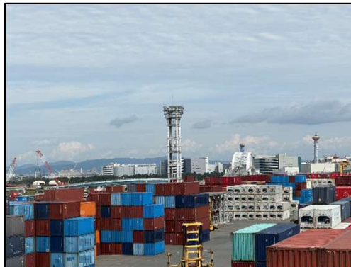
Converting container yard lighting towers to LED
