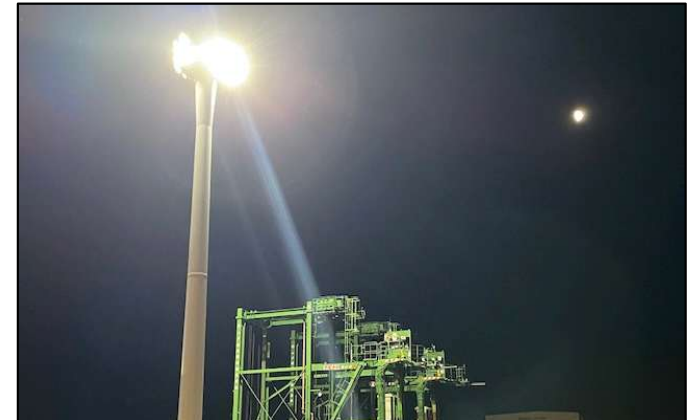
LED conversion of yard lighting
