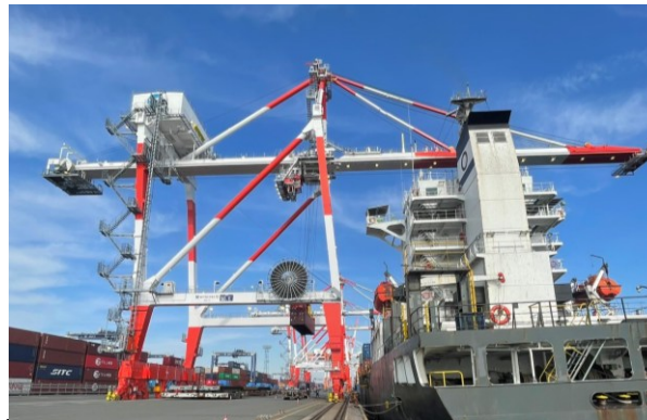
Introduction of inverter-controlled gantry cranes (Newly installed Unit 1)
