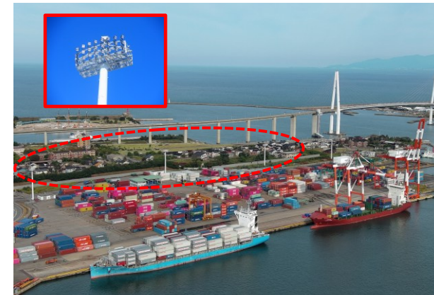
Converting container yard lighting towers to LED
