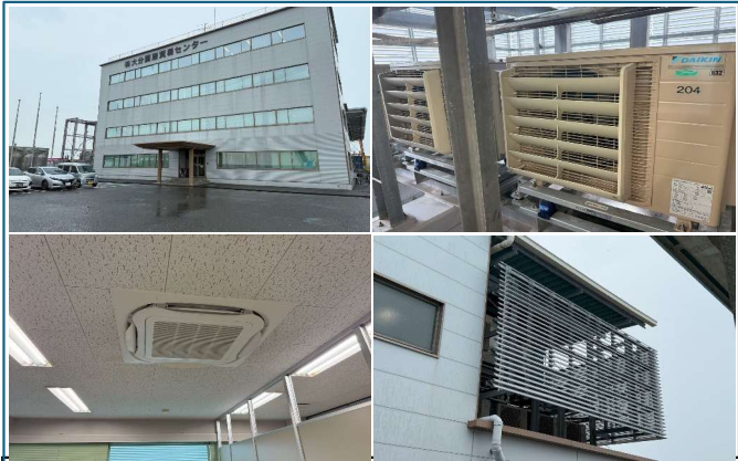
Energy Conservation in the Administration Building(Air-Conditioning System)
