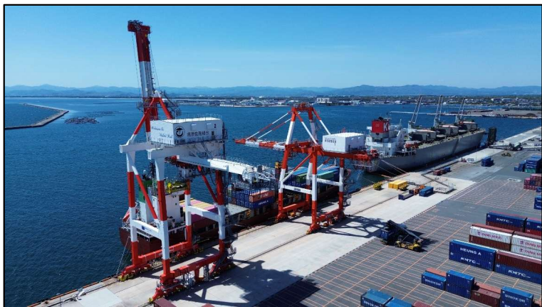
Inverter-controlled gantry cranes (2 units)
