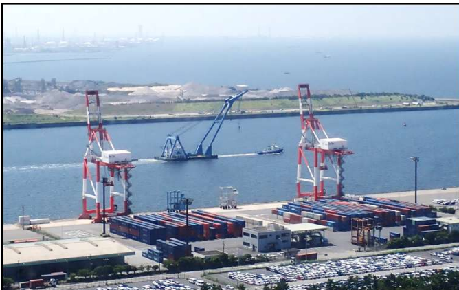
Introduction of gantry cranes with inverter control systems
