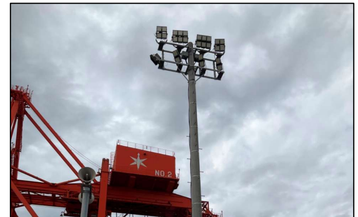
LED conversion of yard lighting
