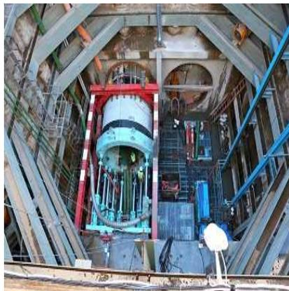
Method to install sewerage pipes without excavating the road (left in the center of photo)
