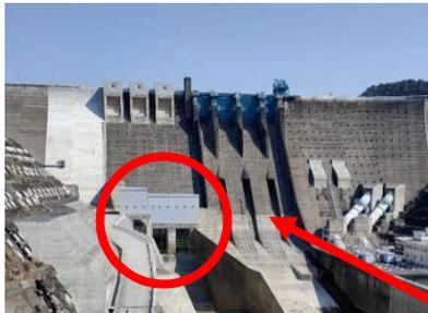
Add a new discharge facility while operating the dam
