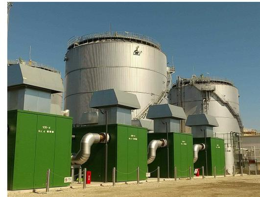
Steel tank in which biogas is generated from sludge and stored (back in the photo) and gas power generator (front in the photo)
