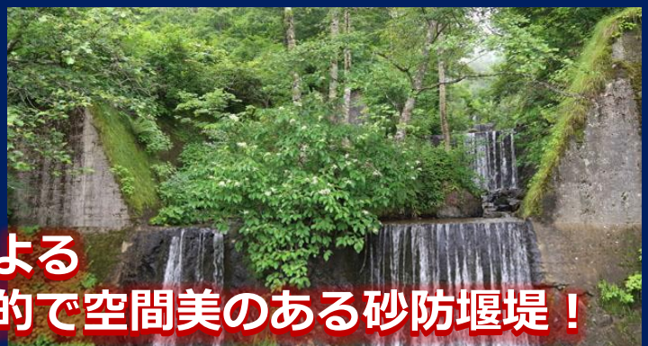
泥谷砂防堰堤
