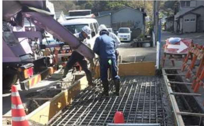
Cast in place concrete manholes
