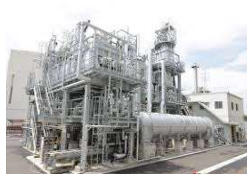
Solid fuel conversion from sewage sludge (Rakusai STP in Kyoto Prefecture )
