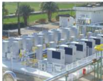
Digestion gas generation facilities (STP in Saga City)
