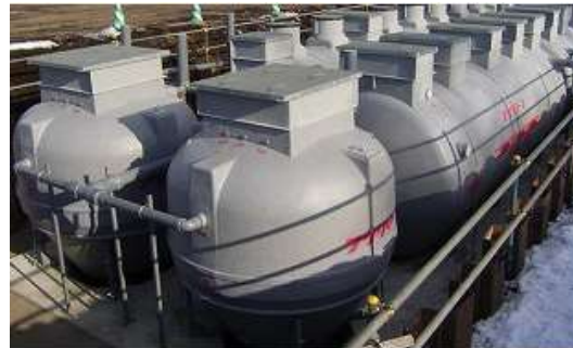
“Quick Project,” which achieves easy construction and low cost by a prefabricated system, is suitable for small-scale WWTPs (Abira-town, Hokkaido)
