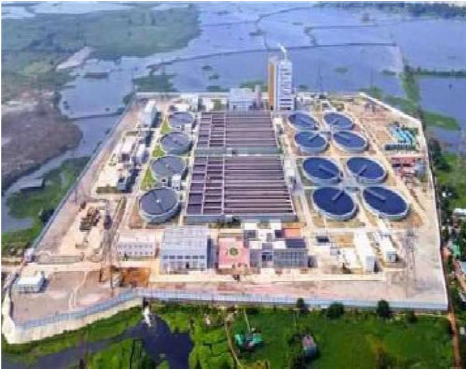
Dasherbandi Sewage Treatment Plant, Dhaka
