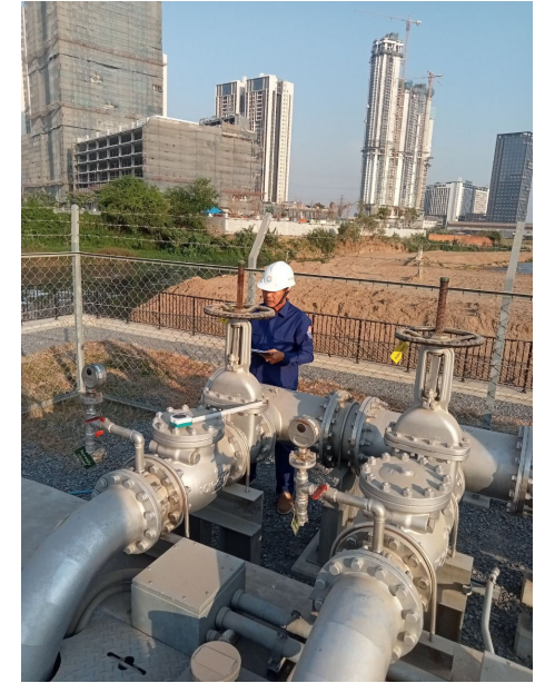
Checking the discharge pressure
