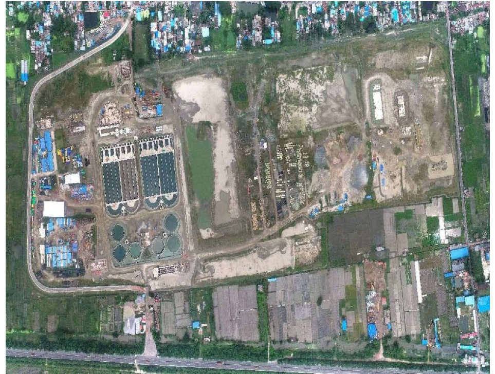
Chattogram Sewage Treatment Plant
