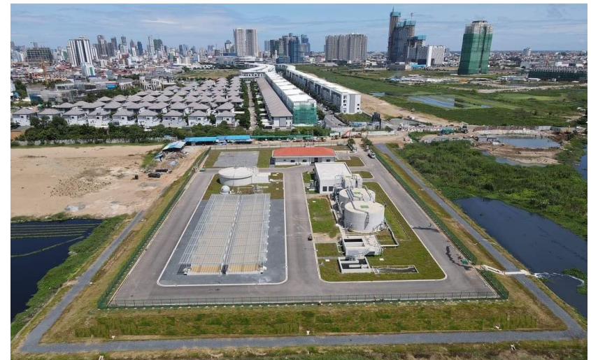
Cheung Aek Wastewater Treatment Plant
