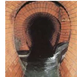
Japan's first modern sewer system Kanda sewer(1884)
