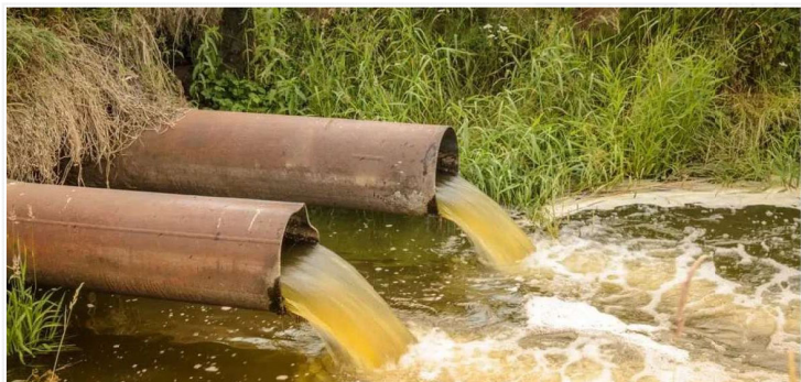
Direct discharge to water source
