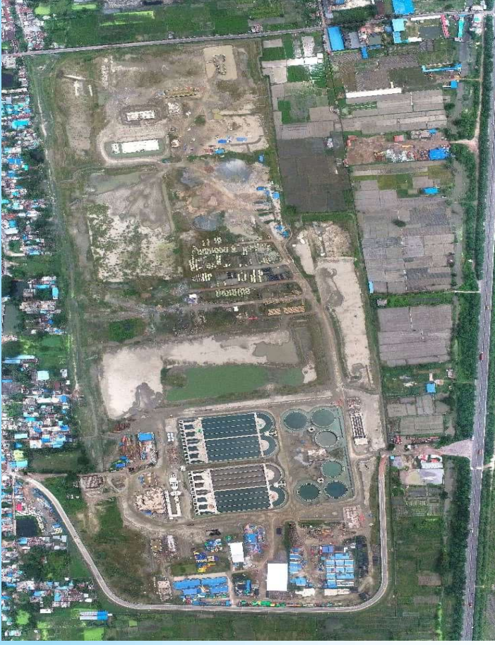
Chattogram Metropolitan Sewerage Project (1 st Phase)
