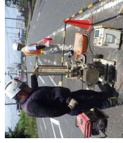
Investigation of the Underground Cavity Below the Road Surface
