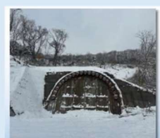
Completion of Construction
