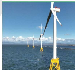
■ Fabrication and Installation of Foundations for Offshore Wind Turbines
