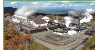
■ Geothermal Power Plants
