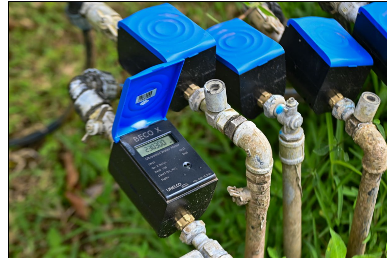
Customer's meter Size 15 and 20 mm
