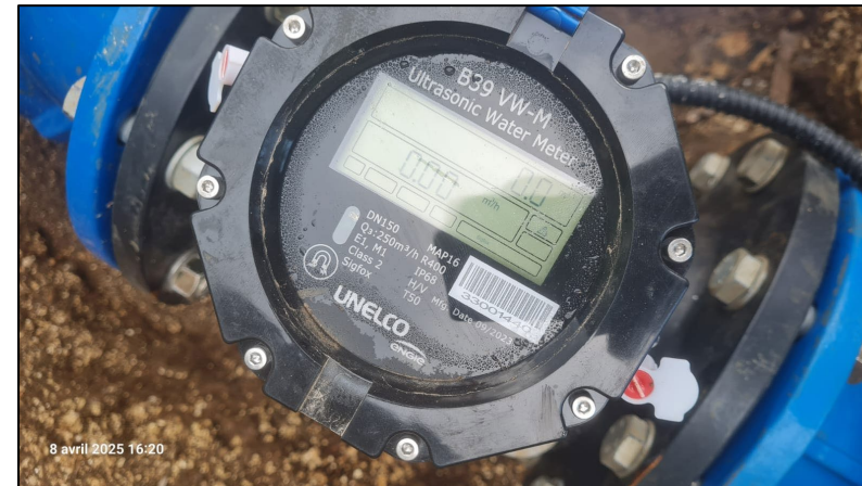
DMA meter or big customer meter (example : resorts)
