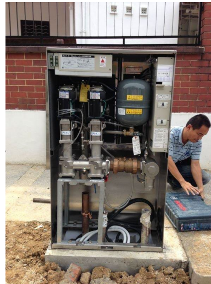
Outer & Inner view of booster system
