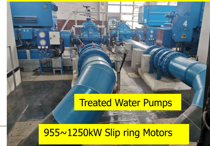
16~21mgdi Horizontal Split Casing pumps, pipeworks & control panels
