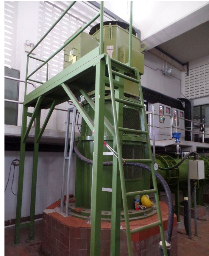
Pump Column 22m long below floor
