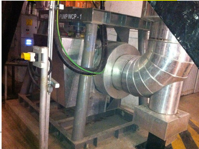
Vertical Split Casing pump
