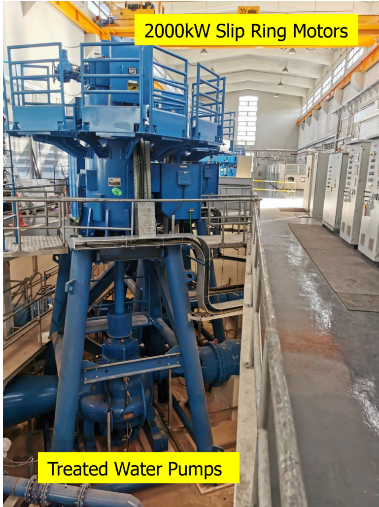
34mgdi Vertical Split Casing pumps & pipeworks
