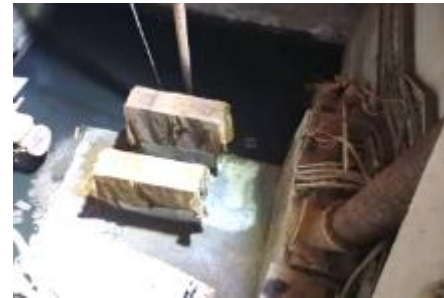
Confirmation of pump foundation construction
