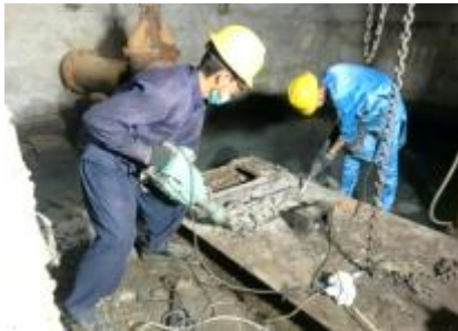
Removal of existing foundation
