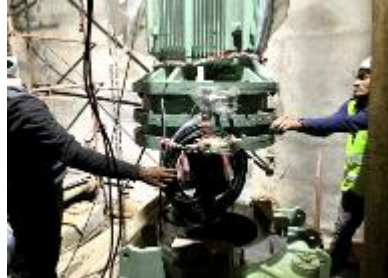
Pump unit installation
