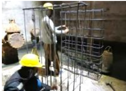
Construction of the pump foundation
