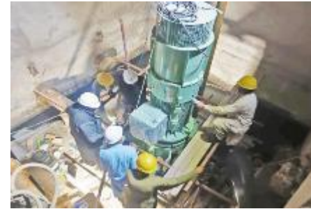
Overview of pump maintenance work
