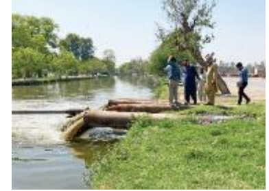
Pump test run
