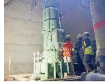
Assembly and installation of the Immersible motor pump are complete.
