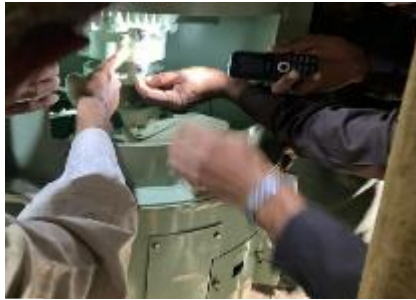
iew of Pump Maintenance Procedures
