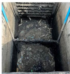
Screen Front Side (sand & debris accumulation)
