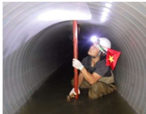
Rehabilitation Pipe (After)
