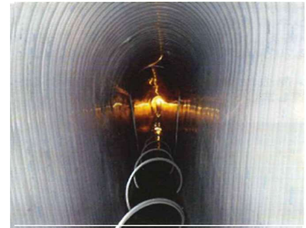
Rehabilitation Pipe (After)
