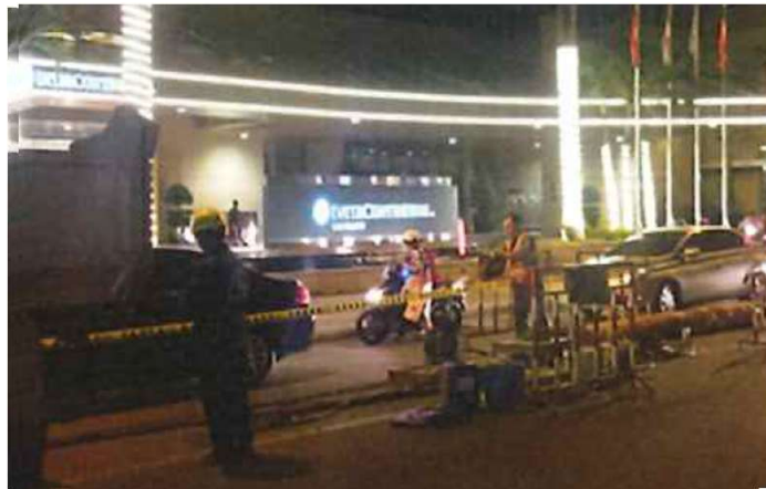
Demonstration Site (Night-time work)
