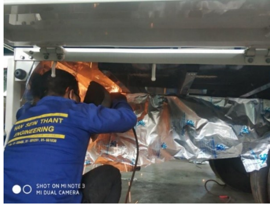
Welding of reinforcing members
