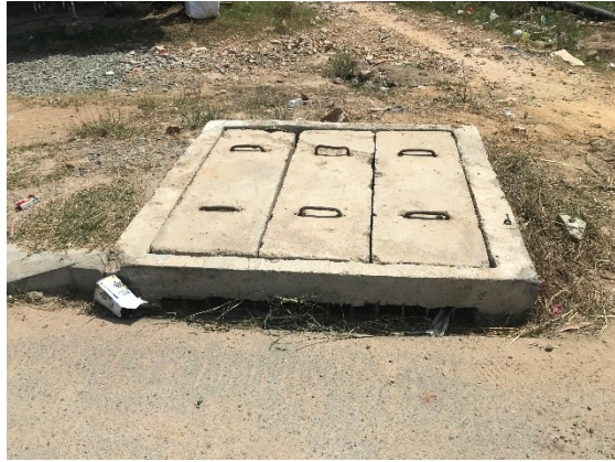
Intake Pump Pit
